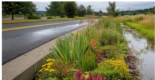
Bioswales are a form of green infrastructure that effectively manage stormwater runoff during storms.
